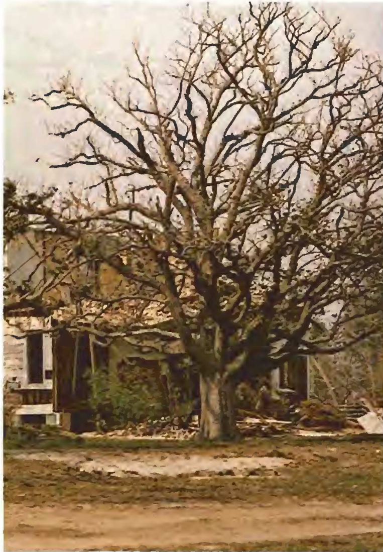
Figure 4. Damaged home and live oak ( Quercus virginiana ) along Highway 90 and open waters of Mississippi Sound at Long Beach, Mississippi.
